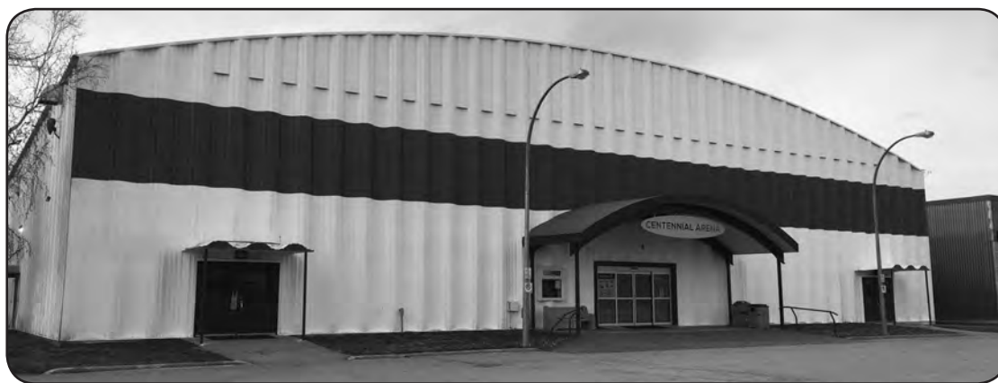
The Winkler Centennial Arena's ice plant gave up the ghost last week, forcing the city to shut down the rink while a new ice-making machine is installed.
